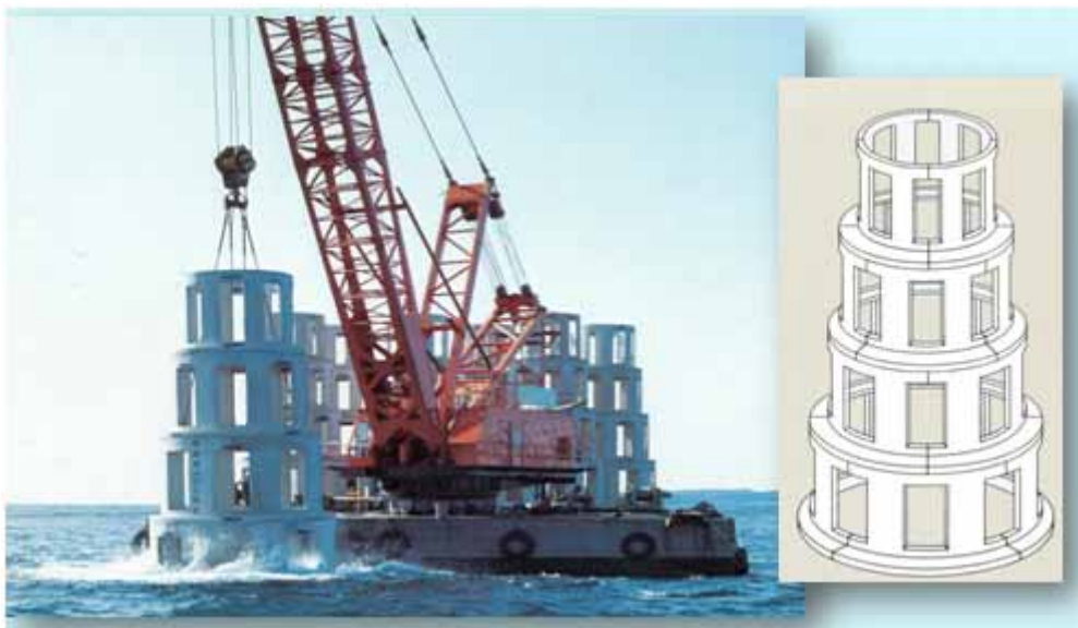
Concrete artificial reef Japan
